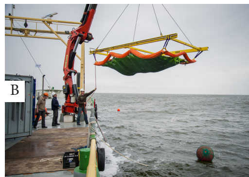
Figure 30. Preparation of the artificial seagrass on the ship. Photo RCE Maritime Programme (A). The artificial seagrass is deployed on the wreck. Photo RCE Maritime Programme/ Paul Voorthuis (B).
